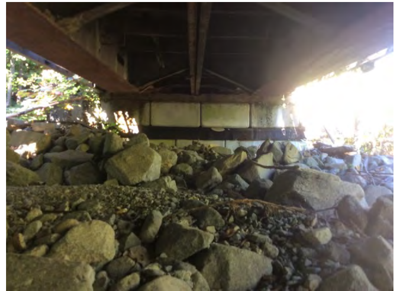
Left Bank Abutment when facing downstream
