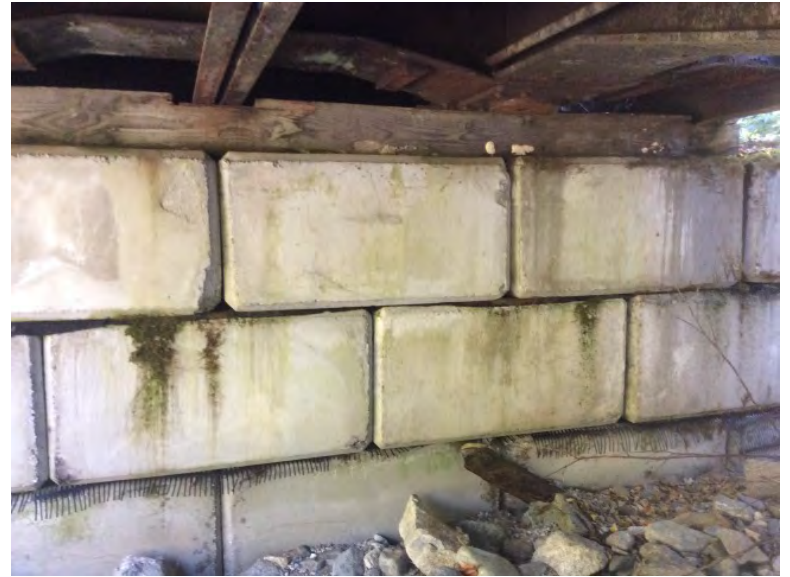
Right Bank Abutment when facing downstream
