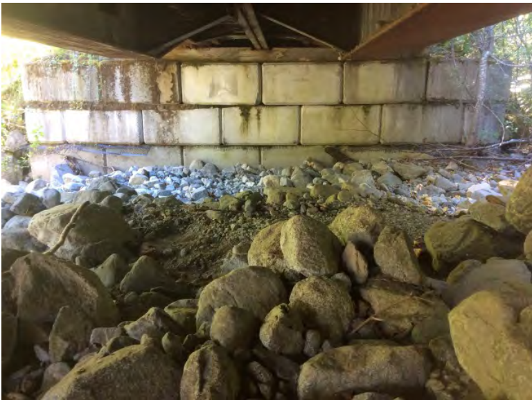
Right Bank Abutment when facing downstream
