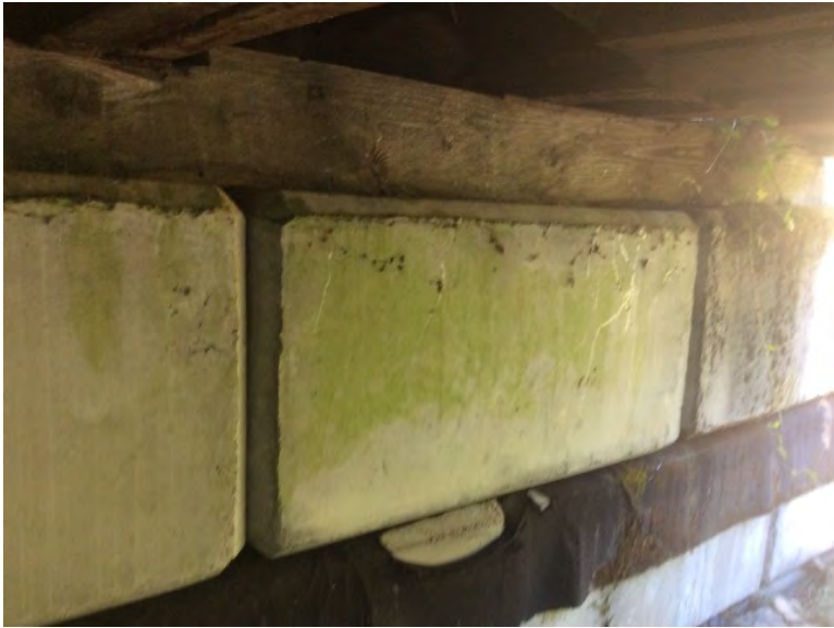
Left Bank Abutment when facing downstream
